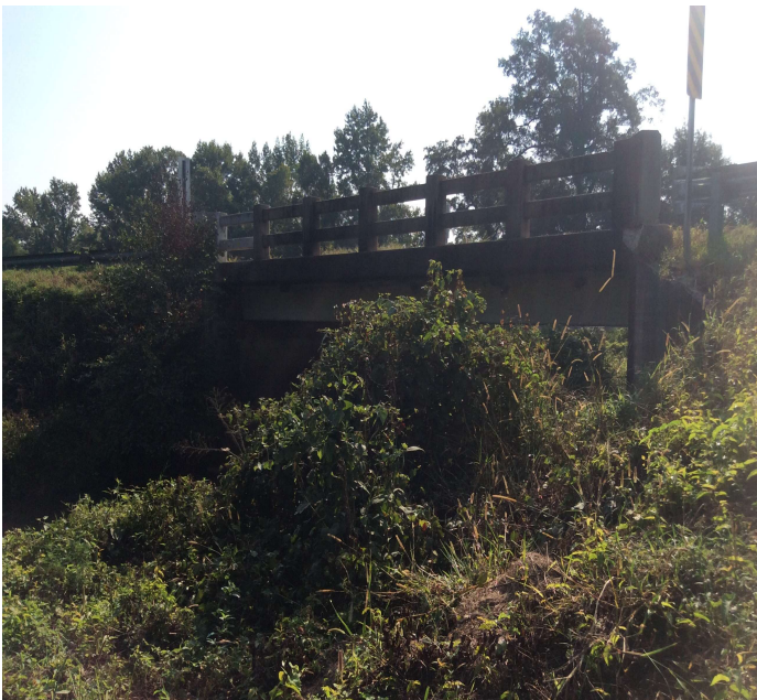
PHOTO 1 Description Small trees, brush and vines growing on and under the bridge.
